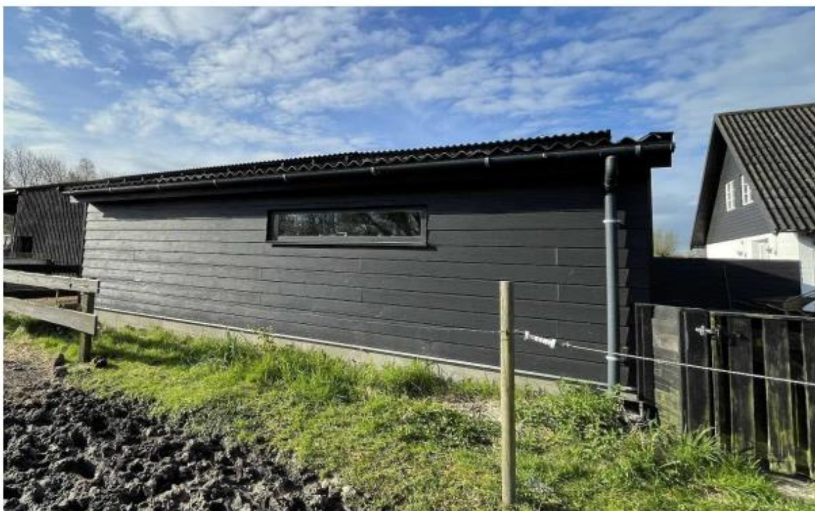
Garage facade mod nord
